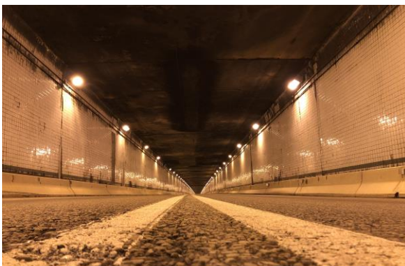
Allegheny Tunnel Somerset County, PA
