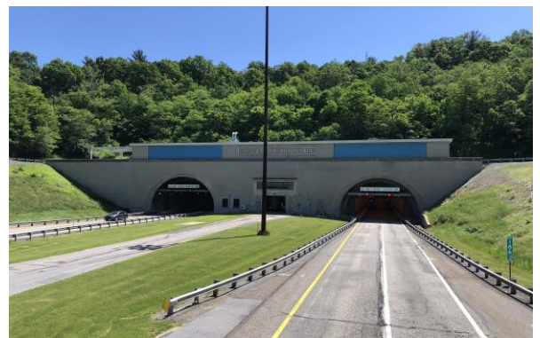
Tuscarora Tunnels Franklin and Huntington Counties, PA
