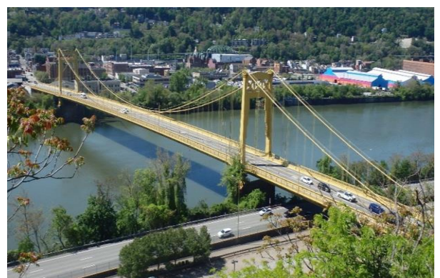
South 10 th Street Bridge
