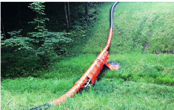
Temporary Waterline Permitting
