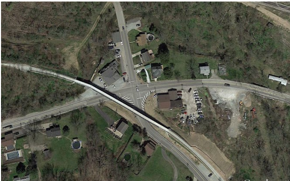
PA 980 Realignment & Pedestrian Bridge
