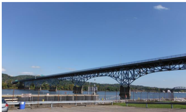
Highland Park Bridge
