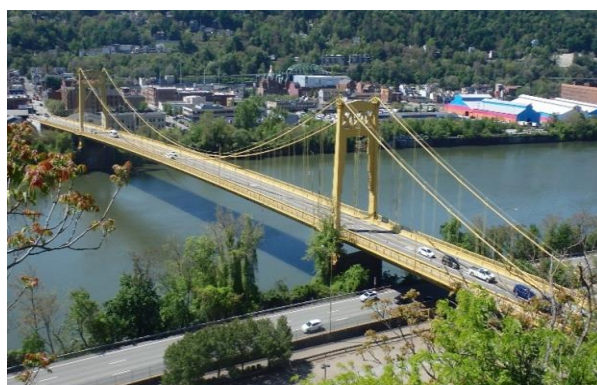
South 10 th Street Bridge
