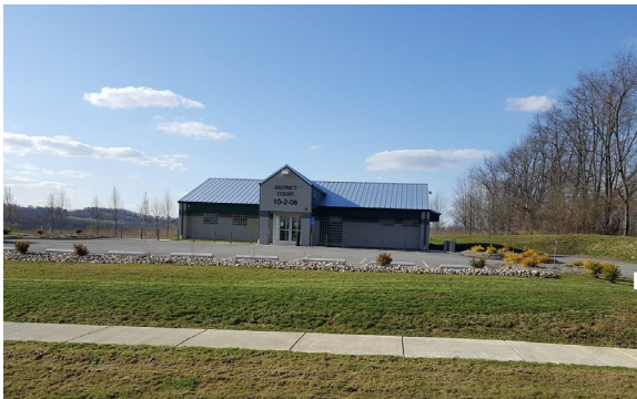
Rostraver Township District Justice Office
