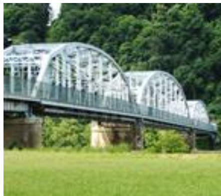
New Kensington Bridge Allegheny County, PA
