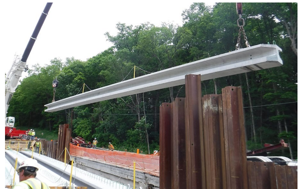
Reidsburg Bridge Clarion County, PA
