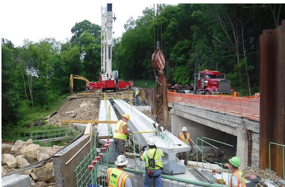
Reidsburg Bridge Clarion County, PA
