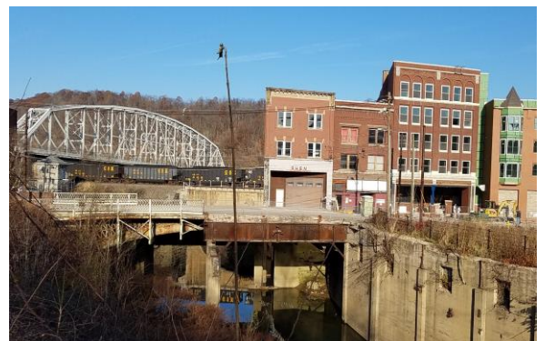
Cast Iron Bridge Rehabilitation Fayette County, PA
