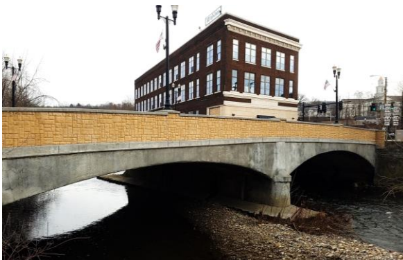
East Washington Street Bridge Lawrence County, PA
