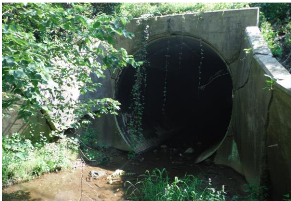
Watters Street Culvert
