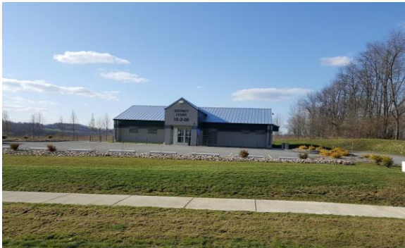
Rostraver Township District Justice Office
