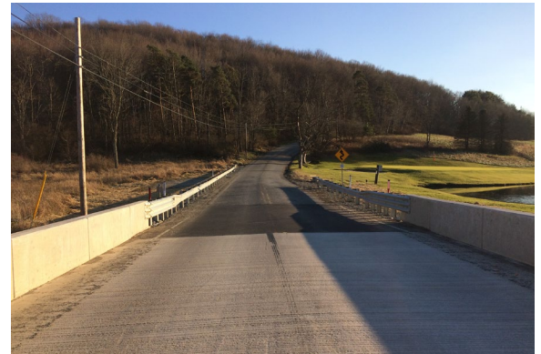
PA Statewide Bridge Replacements – JV 565
