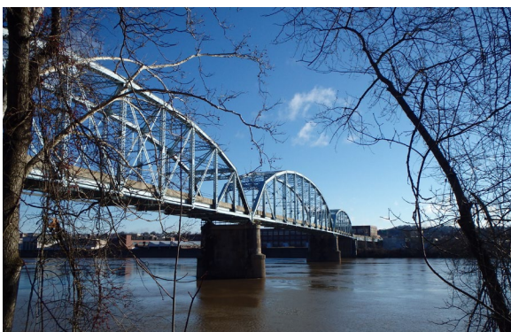
New Kensington Bridge
