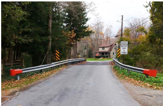
Prefabricated Superstructures – Mill Creek Bridge
