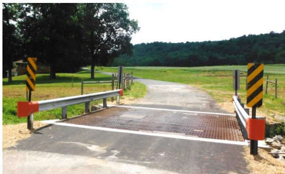
Harvey Road Rhoades Farm Bridge
