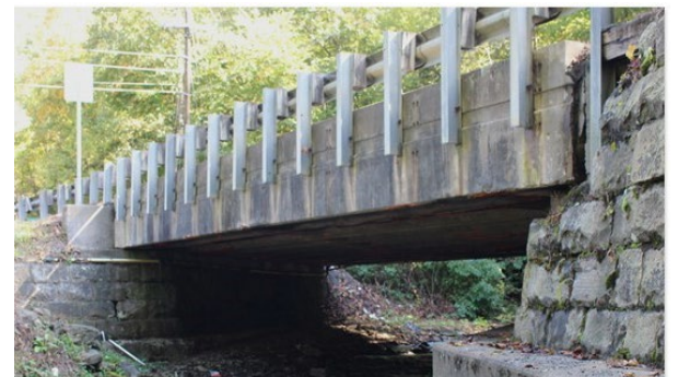
Ralston Branch Bridge
