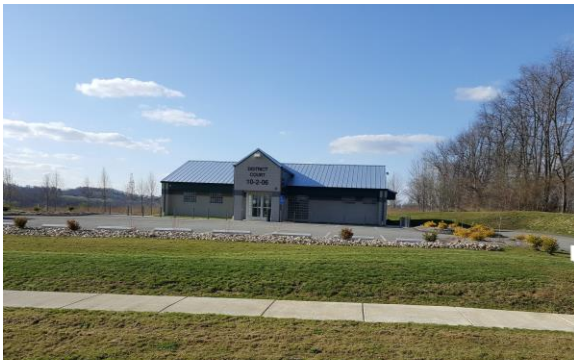
Rostraver Township District Justice Office
