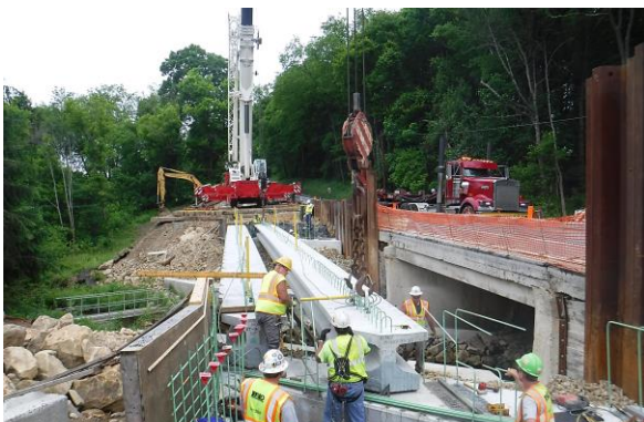
Reidsburg Bridge Clarion County, PA
