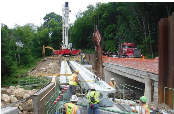
Reidsburg Bridge Clarion County, PA
