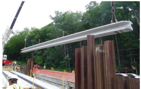
Reidsburg Bridge Clarion County, PA
