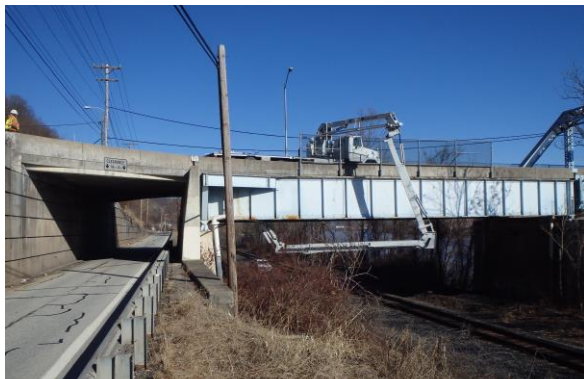
New Kensington Bridge
