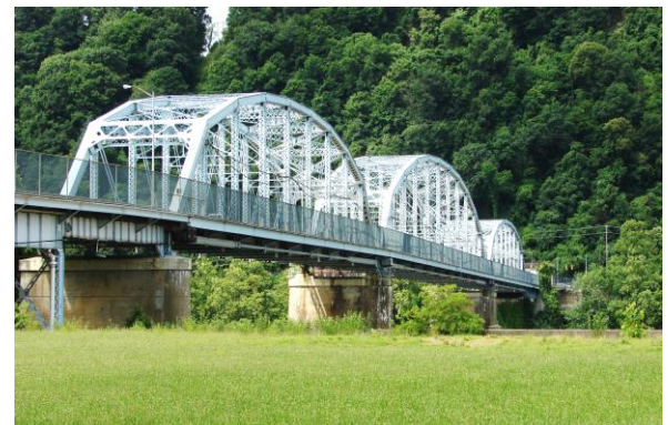
New Kensington Bridge
