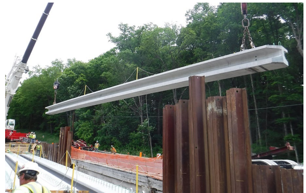
Reidsburg Bridge Clarion County, PA
