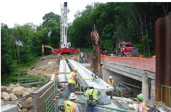
Reidsburg Bridge Clarion County, PA
