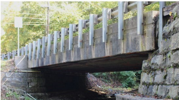
Ralston Branch Bridge
