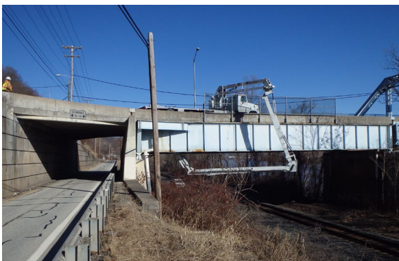
New Kensington Bridge
