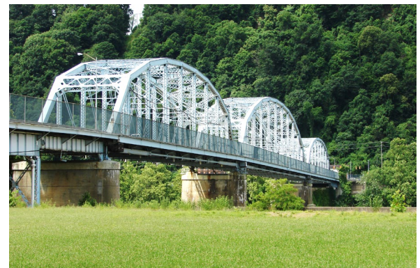
New Kensington Bridge
