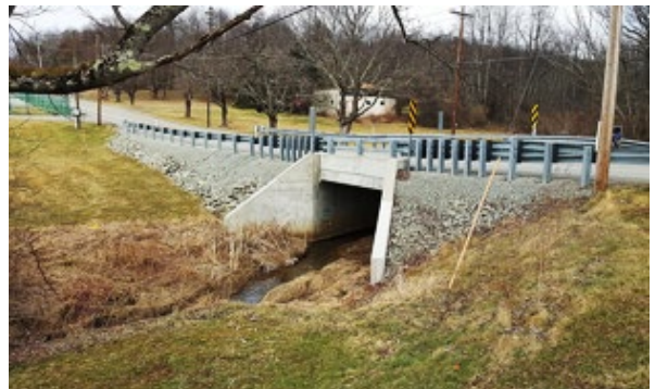
Hills Church Road Bridge
