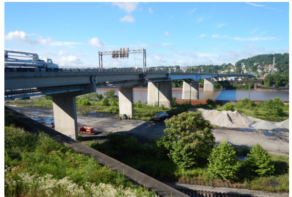
Clairton-Glassport Bridge Allegheny County, PA
