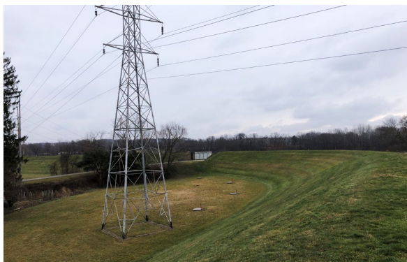
Magnolia Levee Dam Carroll & Stark Counties, OH
