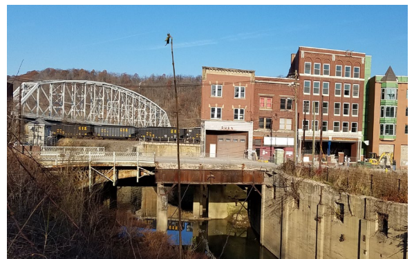
Cast Iron Bridge Rehabilitation Fayette County, PA
