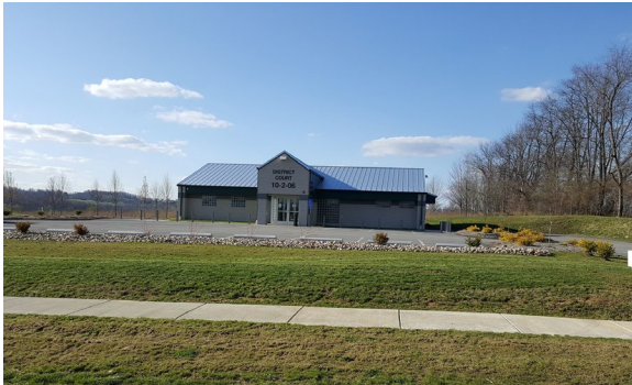
Rostraver Township District Justice Office
