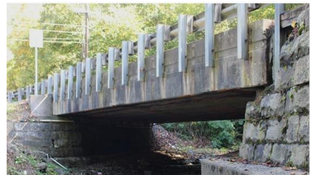
Ralston Branch Bridge
