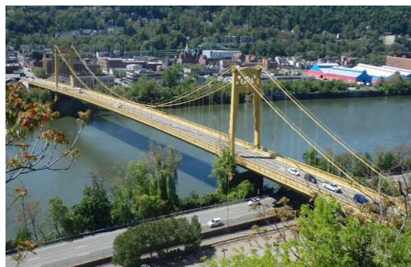
South 10 th Street Bridge
