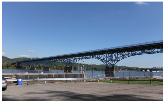
Highland Park Bridge
