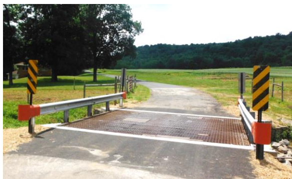
Harvey Road Rhoades Farm Bridge
