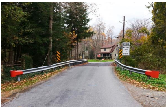
Prefabricated Superstructures – Mill Creek Bridge
