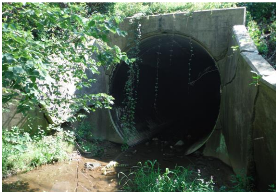
Watters Street Culvert
