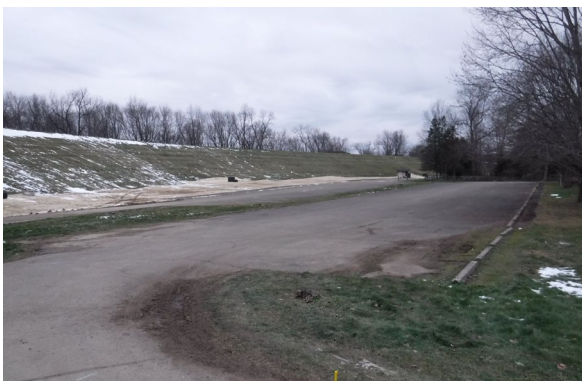
Zoar Levee and Diversion Dam
