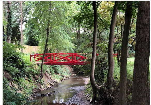
East 20 th Street Bridge
