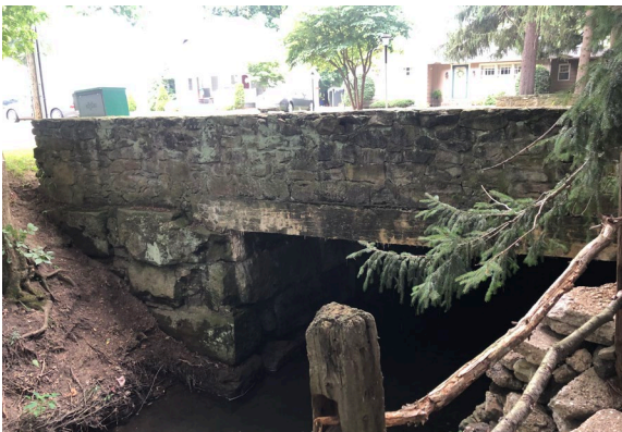
East 20 th Street Bridge
