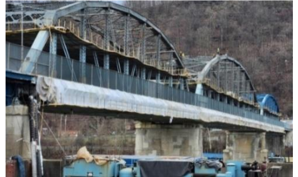
New Kensington Bridge
