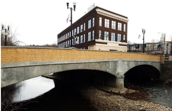
East Washington Street Bridge Lawrence County, PA
