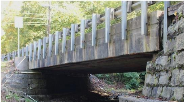
Ralston Branch Bridge
