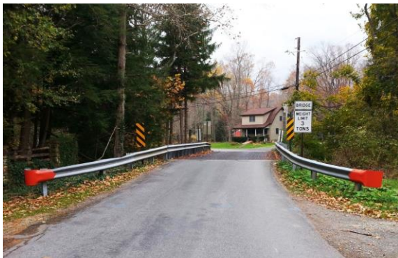
Prefabricated Superstructures – Mill Creek Bridge
