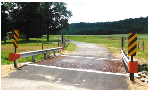
Harvey Road Rhoades Farm Bridge
