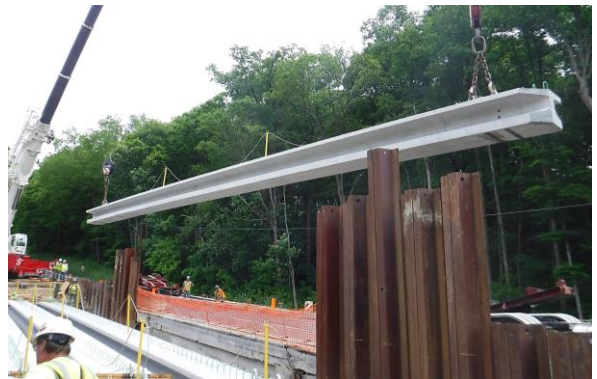
Reidsburg Bridge Clarion County, PA
