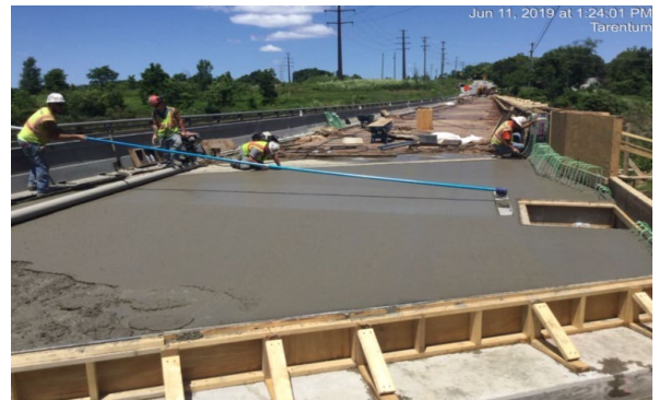
2 Bridges CI – Days Run Road Bridge Allegheny County, PA
