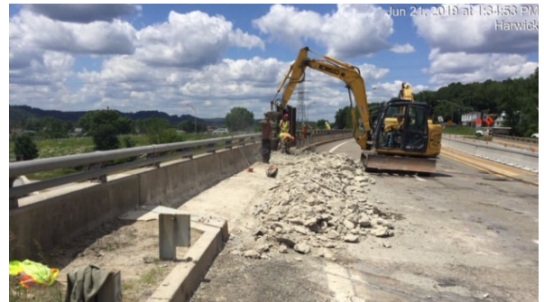
2 Bridges CI – SR 1014 over SR 28 Bridge Allegheny County, PA
