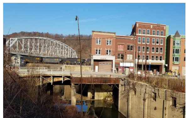
Cast Iron Bridge Rehabilitation Fayette County, PA
