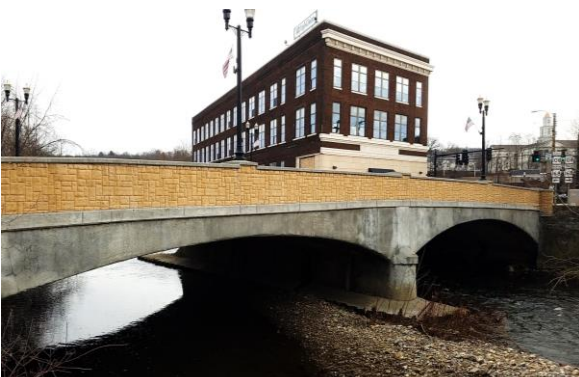
East Washington Street Bridge Lawrence County, PA
