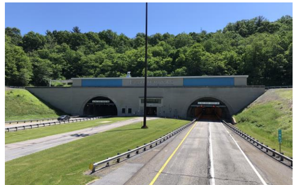
Tuscarora Tunnels Franklin and Huntington Counties, PA
