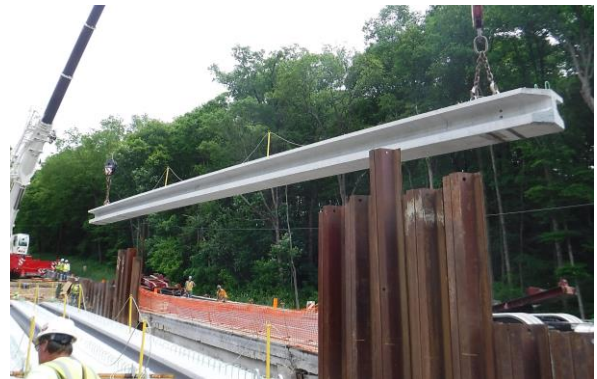
Reidsburg Bridge Clarion County, PA
