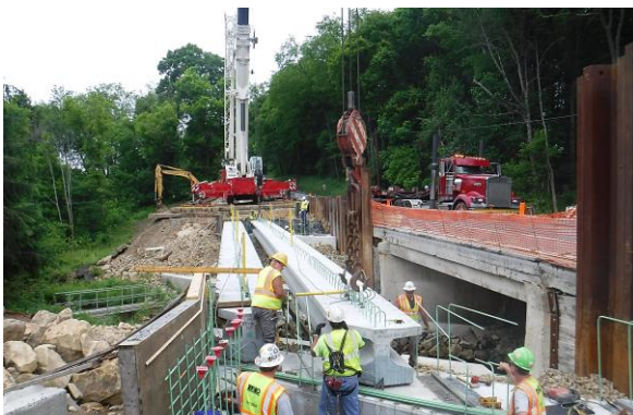
Reidsburg Bridge Clarion County, PA
