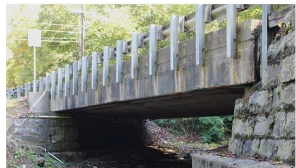
Ralston Branch Bridge
