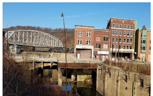
Cast Iron Bridge Rehabilitation Fayette County, PA
