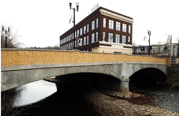
East Washington Street Bridge Lawrence County, PA
