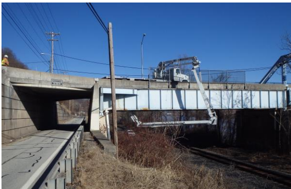
New Kensington Bridge
