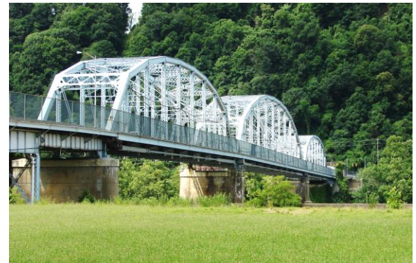
New Kensington Bridge
