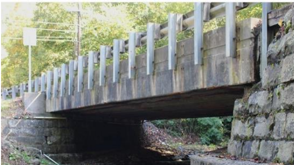
Ralston Branch Bridge
