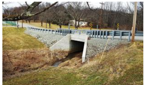
Hills Church Road Bridge
