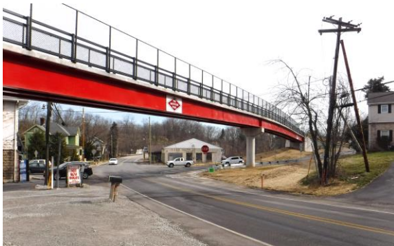
PA 980 Realignment & Pedestrian Bridge
