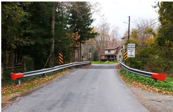
Prefabricated Superstructures – Mill Creek Bridge
