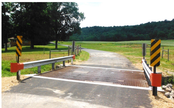
Harvey Road Rhoades Farm Bridge
