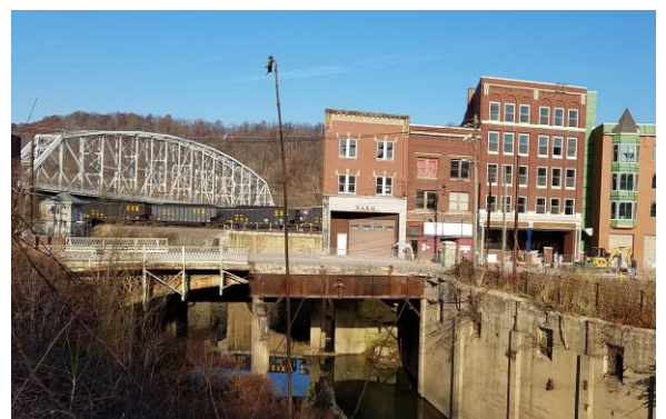
Cast Iron Bridge Rehabilitation Fayette County, PA
