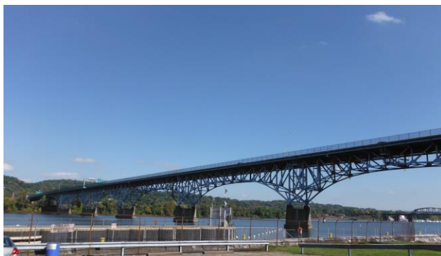
Highland Park Bridge
