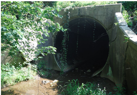
Watters Street Culvert
