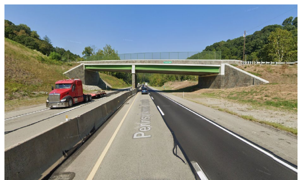
I-76 Trafford Bridge
