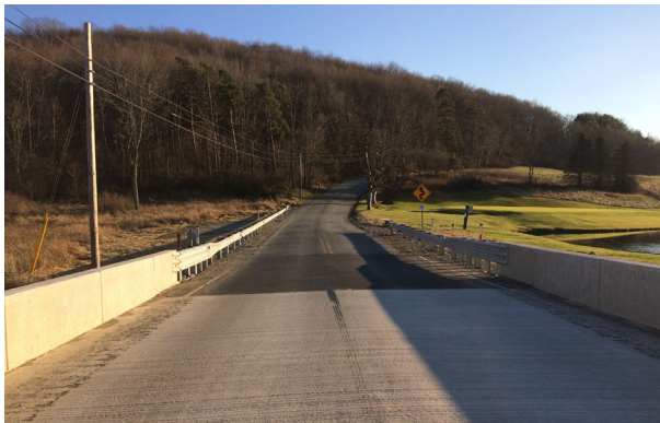
PA Statewide Bridge Replacements – JV 565
