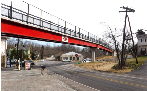
PA 980 Realignment & Pedestrian Bridge
