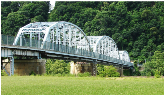
New Kensington Bridge
