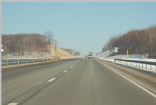
SR 0259, Section 491 Pennview Reconstruction Project
