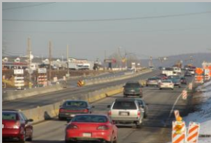
SR 0030 & 0981, Section Q01 Widening and Reconstruction
