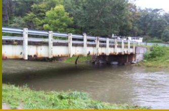
SR 0026, Section 009, PA 26 Yellow Creek Bridge
