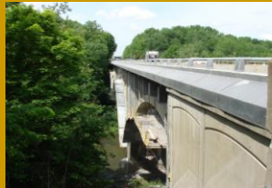
SR 422, Section L12 Rosepoint Bridge Rehabilitation
